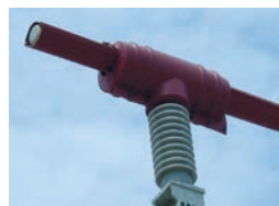
2 Pieces: MVLC-38 on busbar with BCIC
