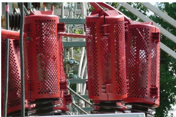
BCAC-IC Installed on Bushings
