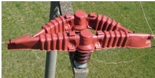
BCIC-1215: Double Post Insulator application
