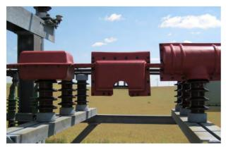
This 20 kV substation in rural Germany is insulated against climbing animals such as martens and cats using wraparound covers that are field cut on site to accommodate any unusual geometry including the center cover where a cut-out has been added to allow access for an earth clamp in a relatively safe position. Covers that need field cutting benefit from being produced from a polymeric cross linked material because they will never propagate splits if they are roughly cut.
