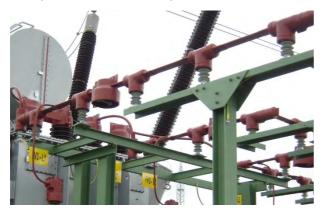
This substation in Croatia shows all bare live metalwork insulated, busbars with heat shrink tubing, connection points with cold applied wrap around covers that can be removed for maintenance or inspection and re-used. The issue was phase to ground clearances on medium voltage side of transformer and bus network where typical 40cm air gaps were being bridged by cats and birds (crows & pigeons).
