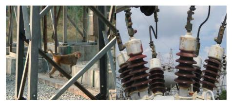
Figure 7. Monkeys in Indian substation and evidence of inter-phase bridging, Greece
