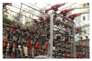
An ageing medium voltage substation in central Athens with huge numbers of cats and pigeons. Many phase to ground clearances well below the nominal 40cm distances and previously suffered multiple flashovers. Solution was to cover the vulnerable bare metalwork with a range of high performance polymeric covers, wraparound sleeking and circular barriers that prevent cats climbing over the insulator and being able to touch Medium Voltage and ground at the same time.
