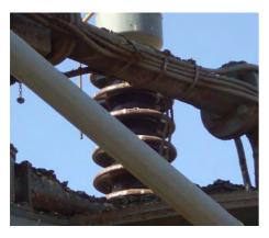
Figure 3. Guano build-up on suspension insulator and on substation equipment.
