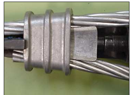
Step 3) Put connector in position guarantying that actuator screw is centralized and perpendicular to Wedge's back face.
