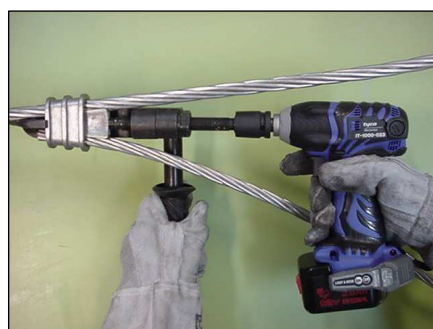
Step 5A) Fit the appropriate socket (n°19 - mm) in the electrical tool for the application and join it to actuator screw.
